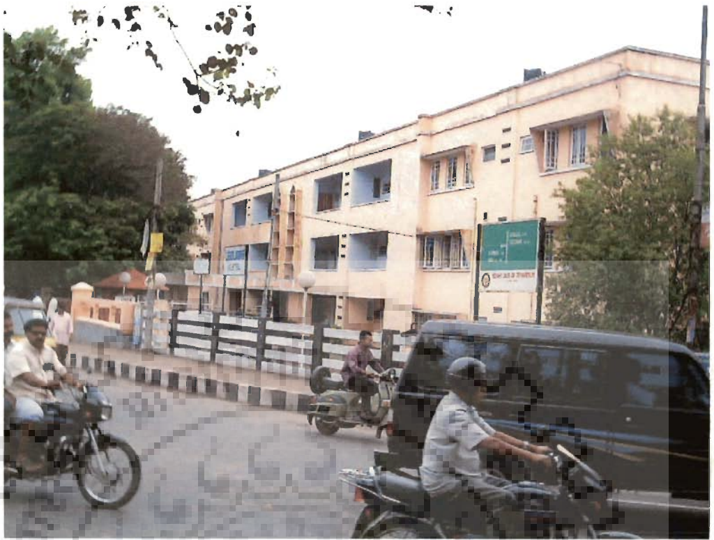
Fig 2. LEGISLATORS' HOSTEL, THIRUVANANTHAPURAM.
