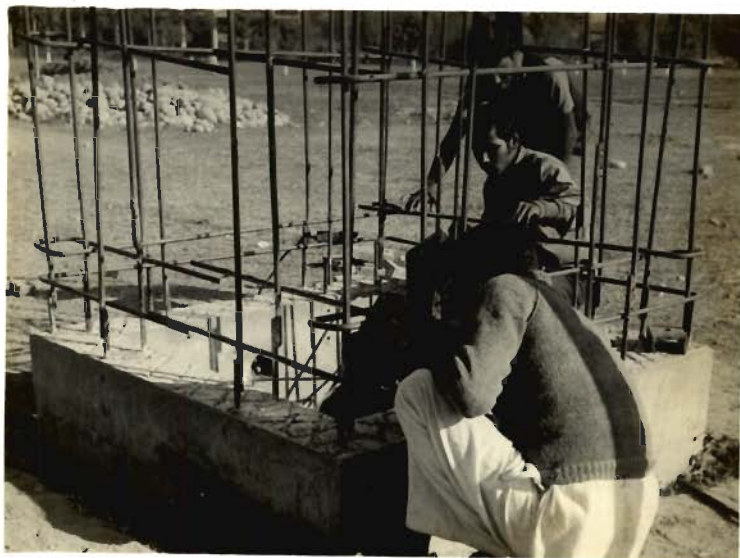
FIG.33-Welding Reinforcement for Third Stage of Steining
