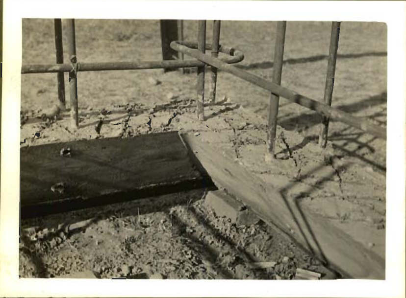
FIG.30-The Concrete Curb and the Cutting Edge
