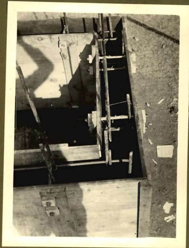
FIG.32-Form-work in Position For First Stage of Steining
