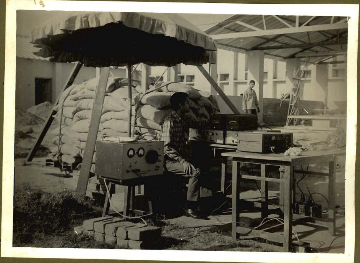
FIG.41-Free Vibration Test in Progress
