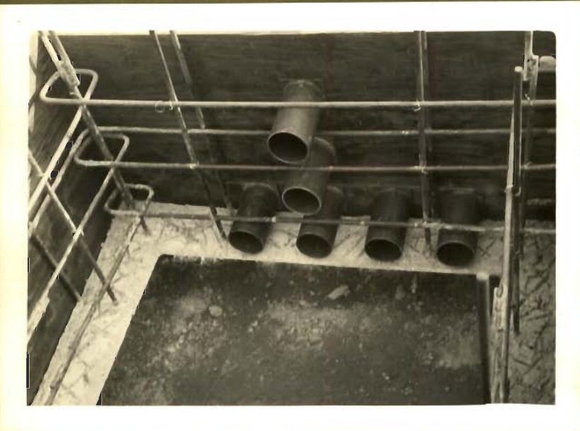
FIG.36-Pipes Screwed to Outer Formwork
