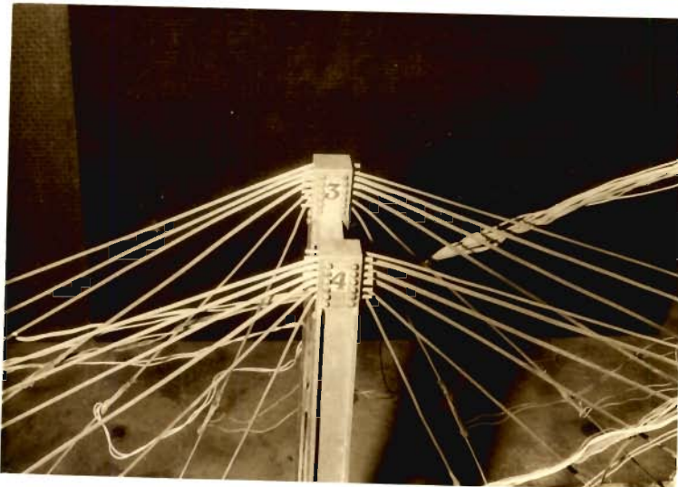
P 6: CABLE ANCHORAGE BLOCKS AT THE TOWER TOP
