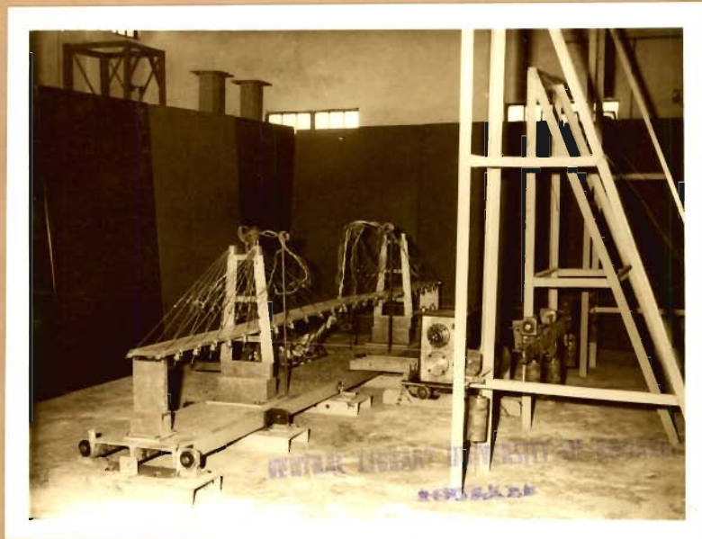
P9: 5-POINT LATERAL LOADING OF THE BRIDGE DECK
