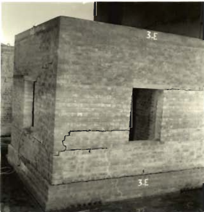
PHOTO 5.36 _ MAINLY HORIZONTAL CRACKS IN EAST CROSS - WALL (MODEL 3 )
