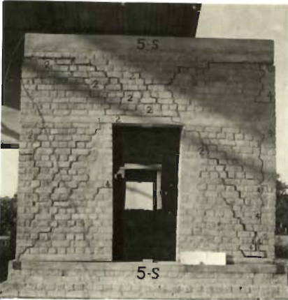
PHOTO 5-81-SEPARATION OF EAST WALL INITIATED AT SOUTH-EAST CORNER (MODEL 5)
