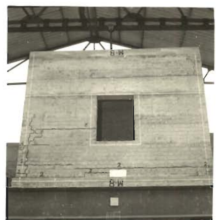
PHOTO 5.125_ HORIZONTAL AND VERTICAL CRACKS IN WEST WALL ( MODEL 8 )
