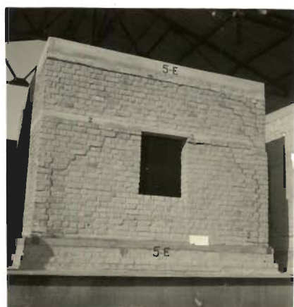
PHOTO 5.79 FEW HORIZONTAL AND DIAGONAL CRACKS IN EAST WALL (MODEL 5)
