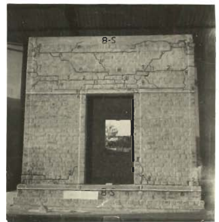
PHOTO 5.134 _ WIDE OPEN CRACK BELOW PLINTH BAND OF SOUTH WALL DURING SHOCK NO. 8 (MODEL 8 )
