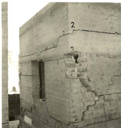
PHOTO 5.97 _ SOUTH WALL DIVIDED INTO LARGE CHUNKS, MOVED FROM THEIR POSITION (MODEL 6)
