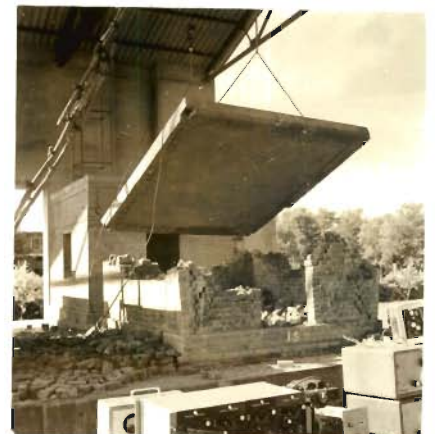
PHOTO 5.17 _ ROOF SLAB LIFTED OFF (MODEL 1)
