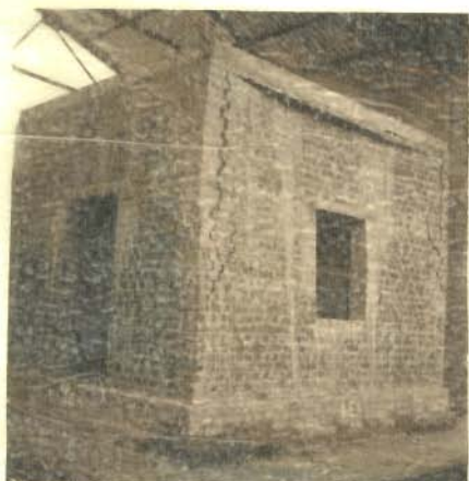
PHOTO 5.12 - EAST CROSS-WALL DEFLECTED INWARD AT TOP (MODEL 1)
