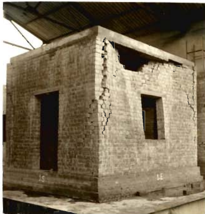
PHOTO 5.13 _ EAST WALL TOP PORTION FELL DOWN (MODEL 1)
