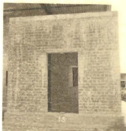
PHOTO 5.11 - VERTICAL AND DIAGONAL CRACKS IN SOUTH SHEAR WALL (MODEL 1)
