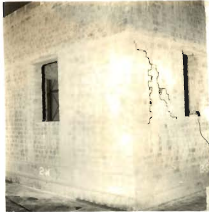
PHOTO 5.19_ VERTICAL AND DIAGONAL CRACKS IN SOUTH SHEAR WALL (MODEL 2)
