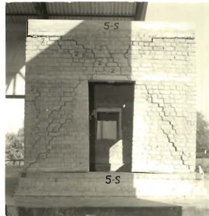
PHOTO 5.77_WELL DISTRIBUTED WIDE CRACKS IN SOUTH SHEAR WALL (MODEL 5)
