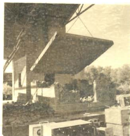
PHOTO 5.17 - ROOF SLAB LIFTED OFF (MODEL 1)
