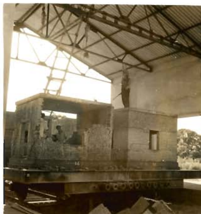
PHOTO 5.16 _MAJOR PORTION OF EAST CROSS- WALL FELL DOWN (MODEL 1)
