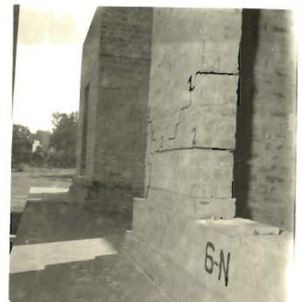
PHOTO 5-89-NORTH SHEAR-WALL PIER BROKEN INTO SEPARATE BLOCKS (MODEL 6)
