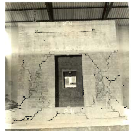
PHOTO 5.26_ SHIFTING OF NORTH - WEST CORNER BOTTOM (MODEL 2)
