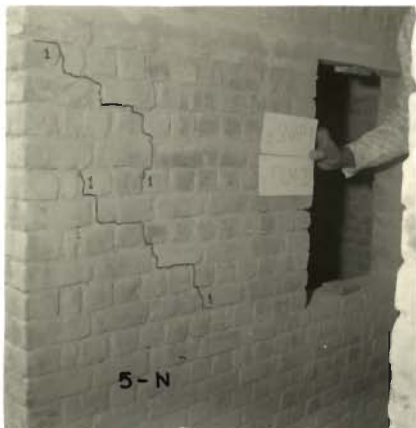
PHOTO 5.72_FINE DIAGONAL CRACKS IN EAST PIER OF NORTH WALL (MODEL 5)
