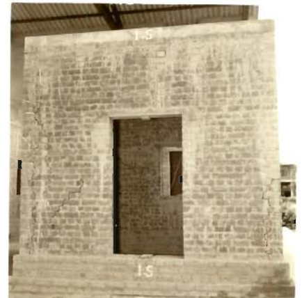
PHOTO 5.11 _VERTICAL AND DIAGONAL CRACKS IN SOUTH SHEAR WALL (MODEL 1)
