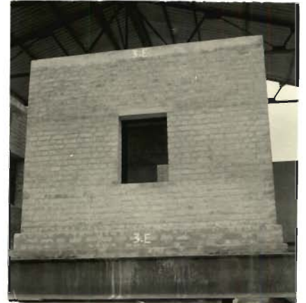
PHOTO 5.31_ INITIAL CRACKS IN EAST CROSS - WALL ( MODEL 3 )
