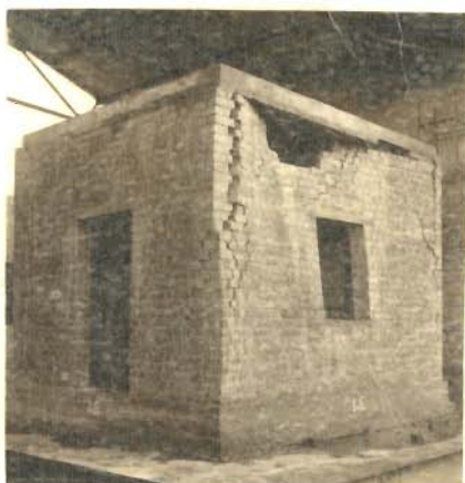
PHOTO 5.13 - EAST WALL TOP PORTION FELL DOWN (MODEL 1)
