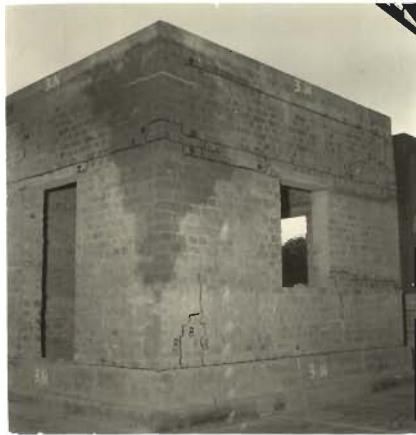
PHOTO 5.40_ VERTICAL AND HORIZONTAL CRACKS IN NORTH AND WEST WALLS ( MODEL 3 )
