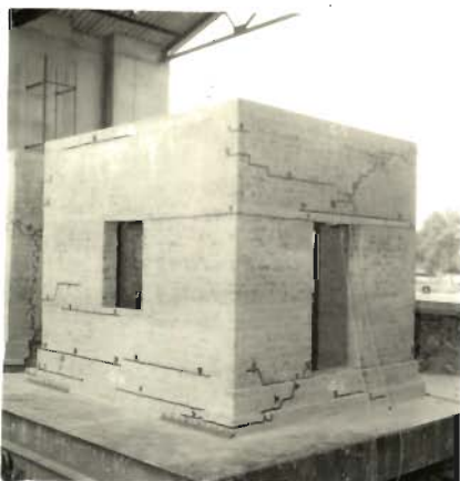
PHOTO 5.54 _ FEW VERTICAL AND MOSTLY HORIZONTAL CRACKS IN WEST WALL (MODEL 4)
