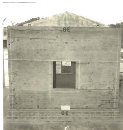
PHOTO 5.124 _ VERTICAL AND HORIZONTAL CRACKS IN EAST WALL ( MODEL 8 )
