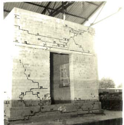
PHOTO 5-68-SOUTH-WEST CORNER SHIFTED OUTWARD (MODEL 4)
