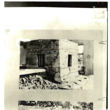
PHOTO 5-71-NORTH SHEAR-WALL AT THE VERGE OF COLLAPSE (MODEL 4)
