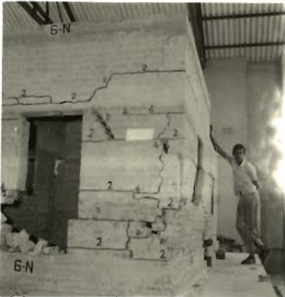
PHOTO 5.99 _ WEST AND NORTH WALLS AT THE VERGE OF COLLAPSE ( MODEL 6 )
