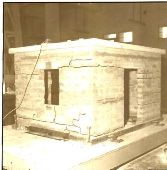
PHOTO 4.5 - DAMAGE TO SOUTH AND WEST WALLS OF MODEL NO. 1 WITH FIXED BASE
