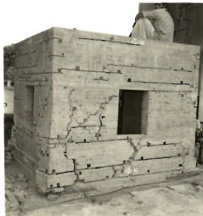
PHOTO 5-70-DIFFERENT DAMAGED PORTIONS OF WEST WALL SHIFTED BODILY CREATING WIDE GAPS BETWEEN THEM (MODEL 4)
