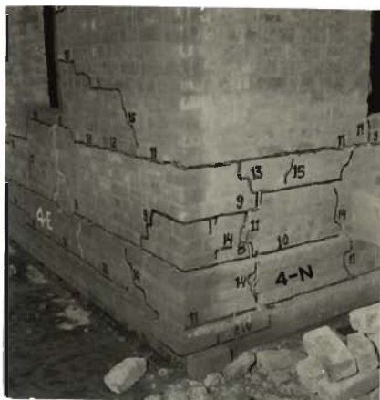
PHOTO 5.58 _ BOTTOM PORTION OF NORTH - EAST CORNER DAMAGED (MODEL 4)
