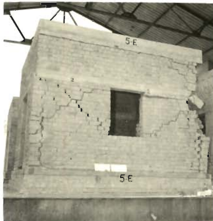
PHOTO 5-85-UPPER PART OF NORTH-EAST CORNER FELL DOWN COMPLETELY (MODEL 5)
