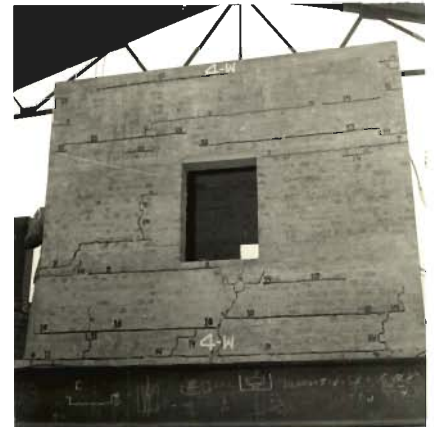
PHOTO 5-65-INITIAL CRACKS (BELOW WINDOW) OPENED UP IN SHOCK NO.15 (MODEL 4)
