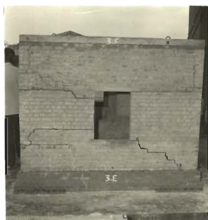
PHOTO 5.43_ MANY CRACKS DEVELOPED IN EAST WALL DURING SHOCK NO.8 (MODEL 3)
