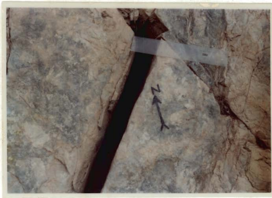
Plate 5.3 Joint opening without filling material
