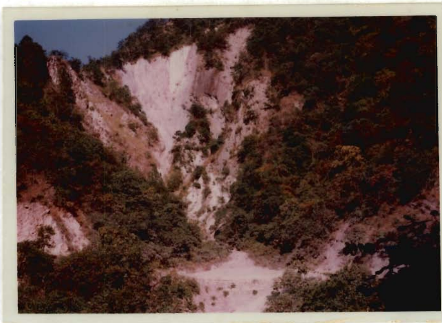
Plate 3.4 Debris slide along a drain
