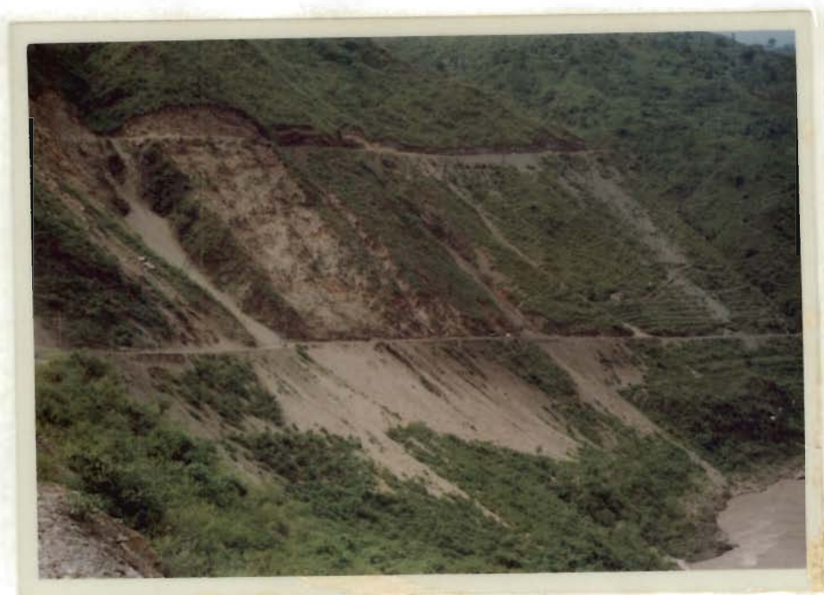
Plate 3.6 Debris flow due to recent road construction
