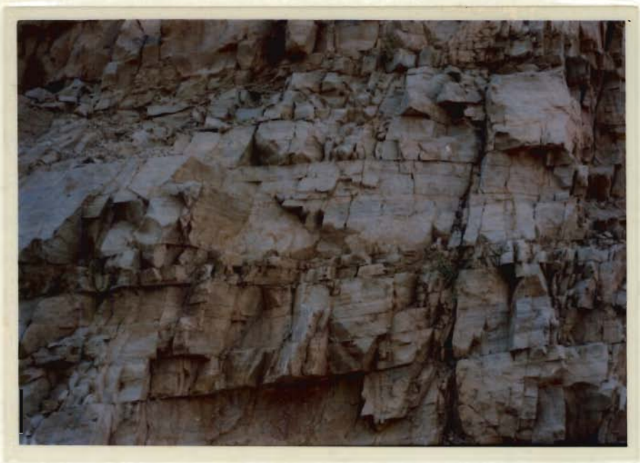
Plate 5.1 Highly jointed quartzite showing low RQD
