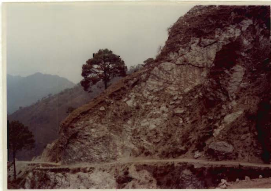
Plate 3.2 Planar failure in phyllite
