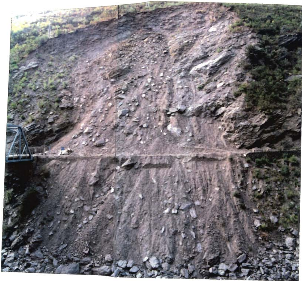
Landslide in phyllites along dam road south of Tehri.
