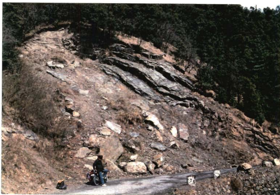
Plane failure in quartzites of Berinag Formation near Surkunda.
