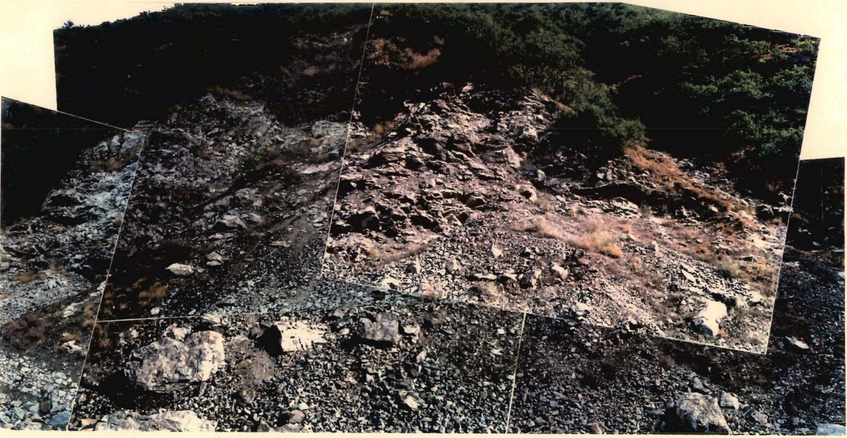
PLATE 5.3 A PART OF KR30A SLOPE SECTION FAILED ALONG ATAL TIUNI ROAD
