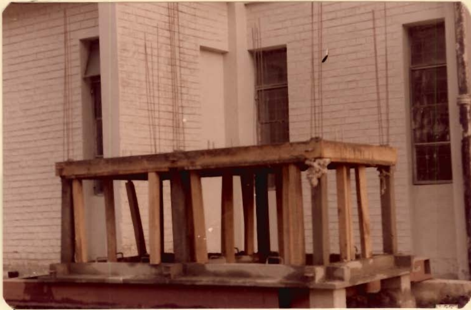
Photo 4.1 : Construction of the Test Structure - Stage I
