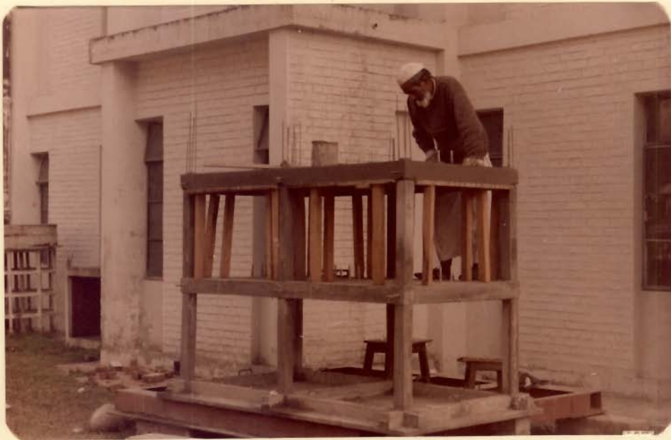
Photo 4.2 : Construction of the Test Structure - Stage II
