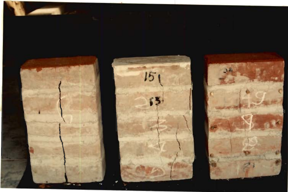
(b) Typical Failure of Masonry Prism under Uniaxial Load
