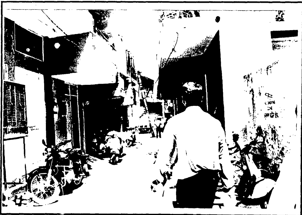
BALCONIES PROJECTED OVER ROAD.
