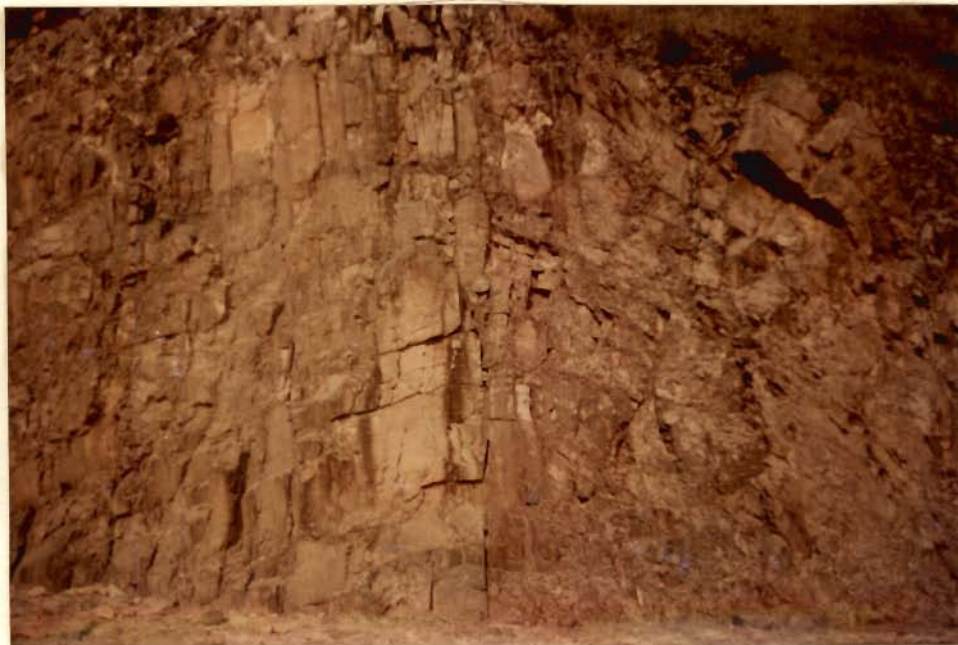
Figure 3.10 (B). Field photograph showing closely spaced fractures in Precambrian folded quartzite. The axis of the fold has been faulted and show numerous fractures. Loc.-29 km south of Shillong towards Pynursla.
