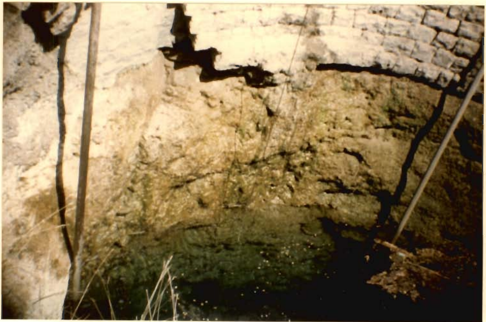
Fig.3.2 : A dugwell tapping highly weathered and fractured non-vesicular massive trap at Yeravle in the lower reaches.
