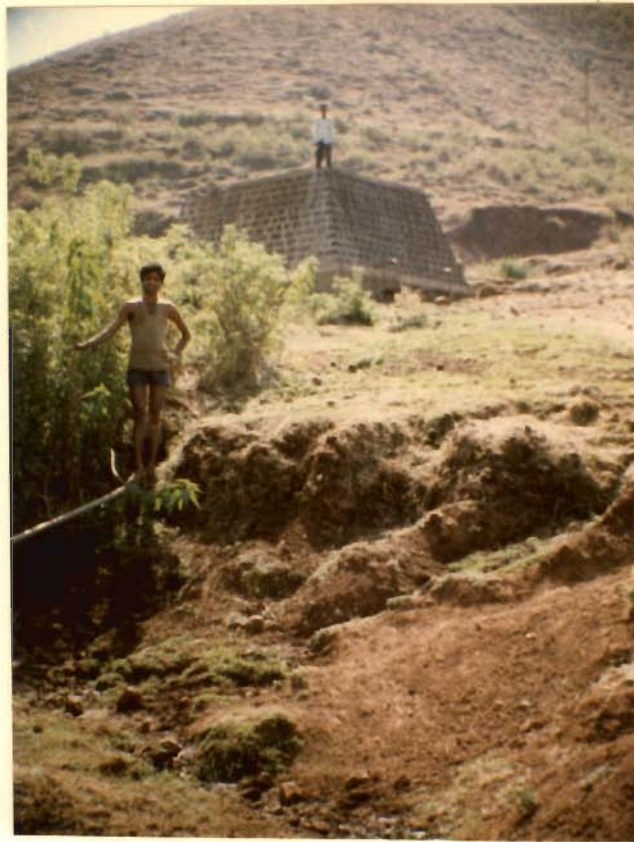
Fig.4.12 : Storage-tank and delivery pipe for storage and supply of spring water.
