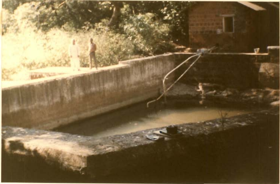
Fig.4.18 : A storage tank constructed by Britishers during pre-independence period for storing spring water and supplying it to their bunglows on hill tops through lift-system (Mahabaleshwar-Spring No.6) (elevation 1240m above MSL).
