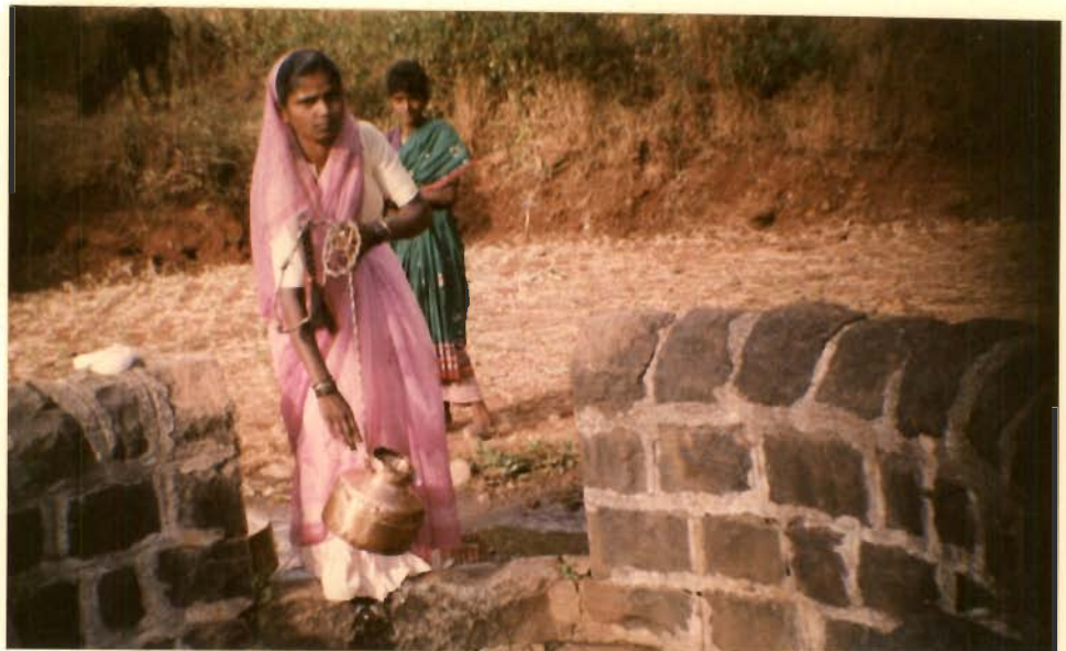
Fig.4.13 : A spring converted into a dug-well at Bhandri (depth of dugwell about 2m ) (elevation 700m above MSL).
