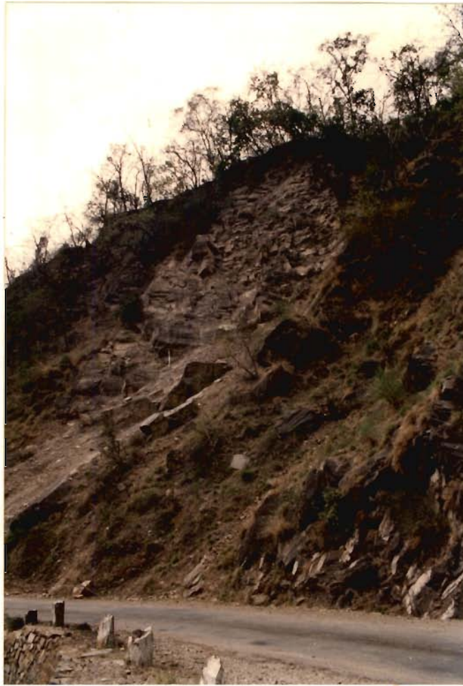
Fig. 5.6 : Wedge Failure in Highly Jointed and Fractured Quartzite (42 km from Rishikesh)
