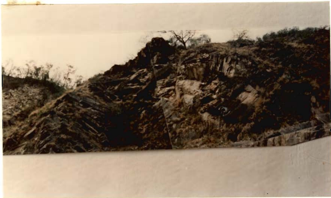
Fig. 5.7 : Occasional Planar Failure in Well Jointed Siltstone (42 km from Rishikesh)
