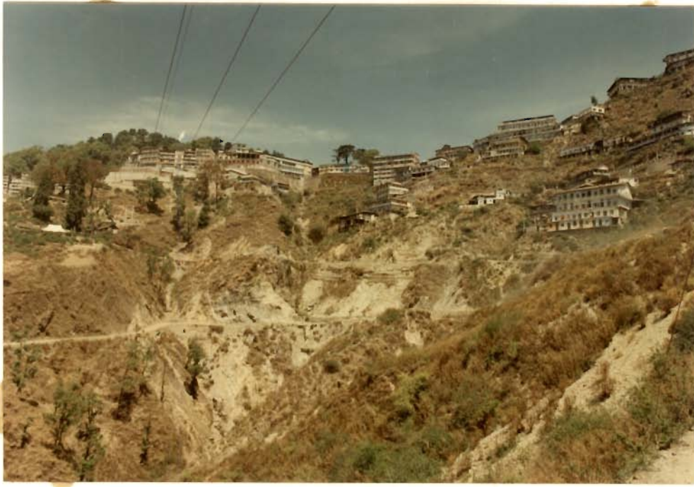
Fig. 4.4 : Panoramic View of Mussoorie Bypass
