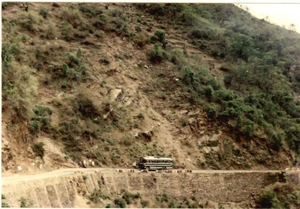
Fig. 3.8 : Rock cum Debris Avalanches in Highly Weathered Phyllite (65 km from Rishikesh)
