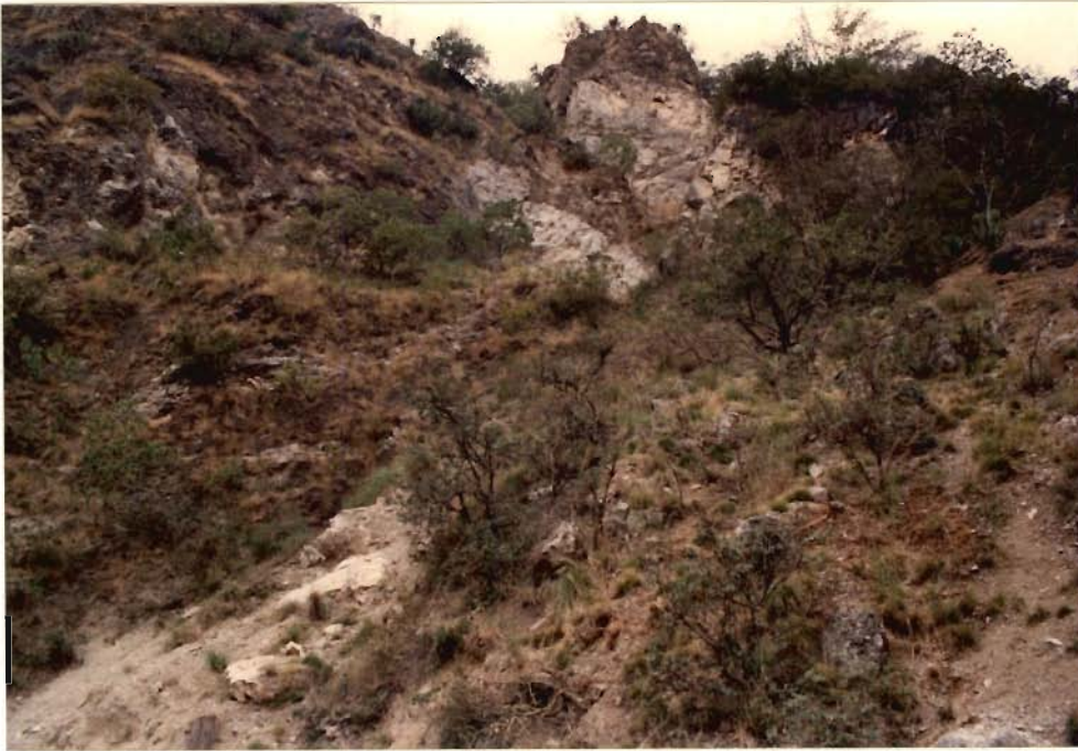
Fig. 5.9 : Rock Avalanches in Jointed and Weathered Limestone (43 km from Rishikesh)
