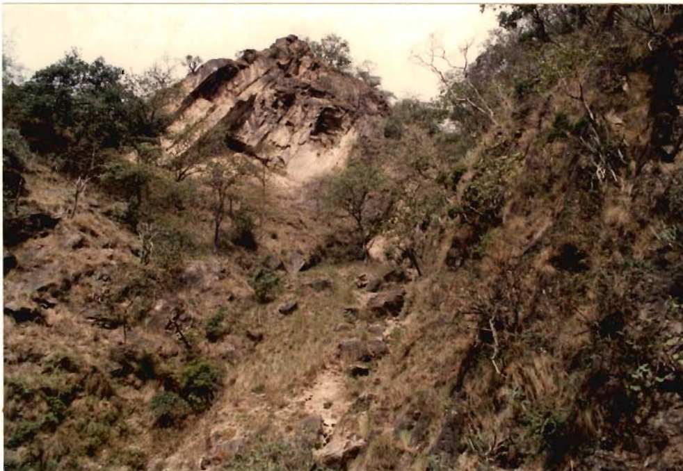
Fig. 5.4 : Occasional Wedge Failure and Rock Fall in Jointed Quartzite (35.3 km from Rishikesh)
