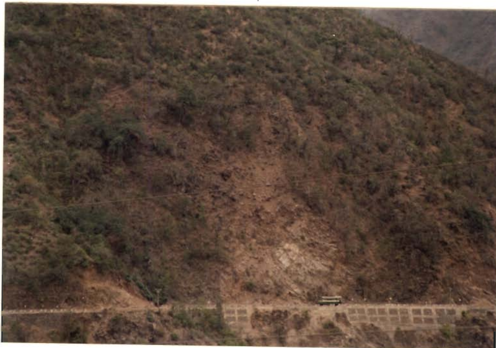
Fig. 5.12 : Planar Slide Cum Debris Avalanches in Well Jointed Quartzite (61 km from Rishikesh)
