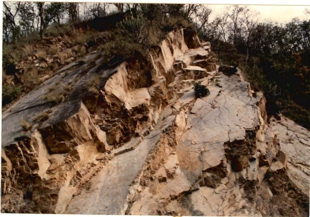
Fig. 5.2 : Planar Slide in Well Jointed and Fractured Quartzite (32 km from Rishikesh)
