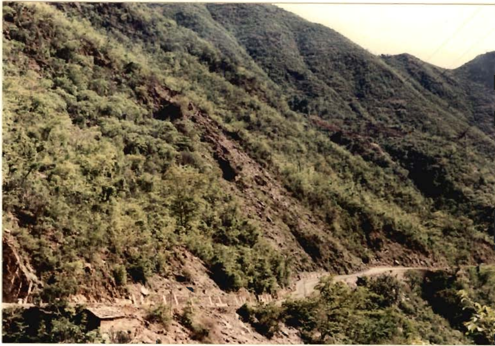
Fig. 5.13 : Debris slide in Weathered Phyllite (65 km from Rishikesh)
