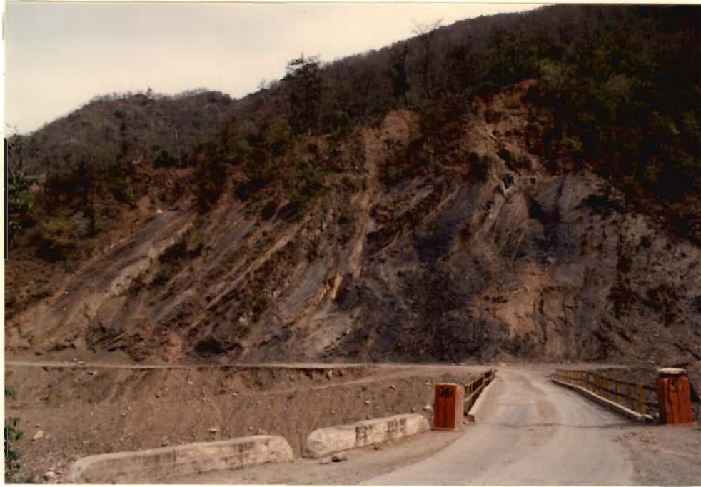
Fig. 3.7 : Rock and Debris Slide in Well Jointed and Weathered Slate (38 km from Rishikesh)
