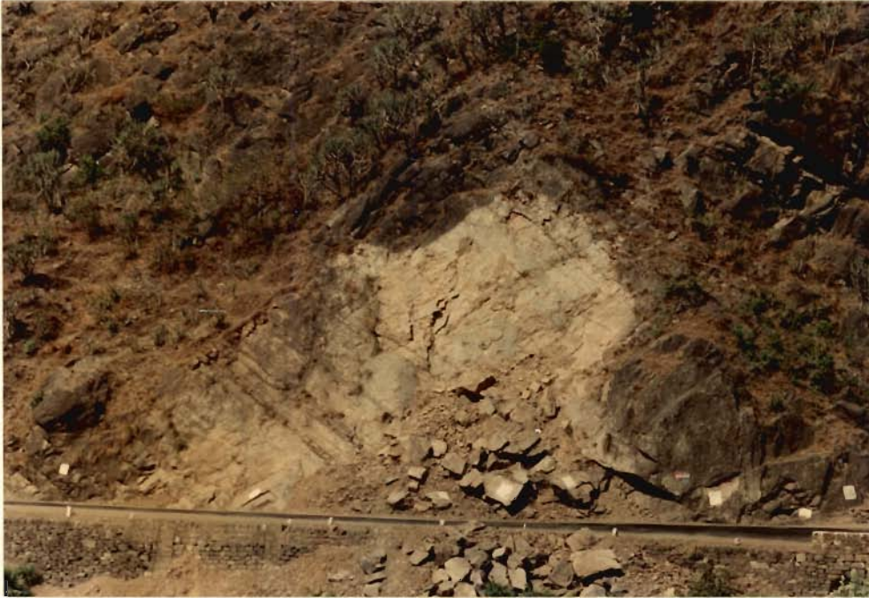
Fig. 5.11 : Wedge Cum Planar Failure in Well Jointed Quartzite (52.5 km from Rishikesh)
