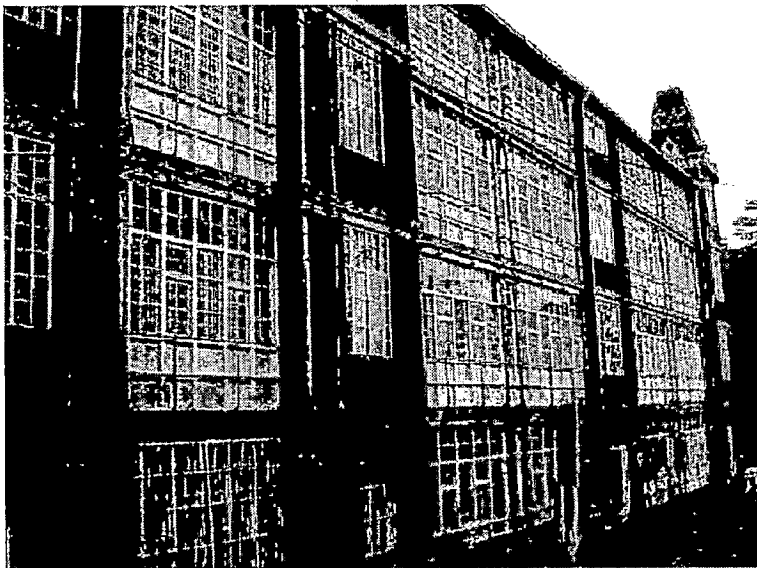
Fig 7.12: Glazed north facade
