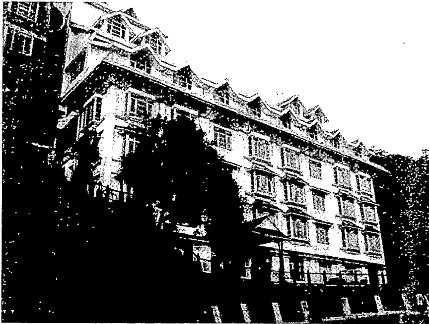
Fig 7.37: Glazing on south facade of building
