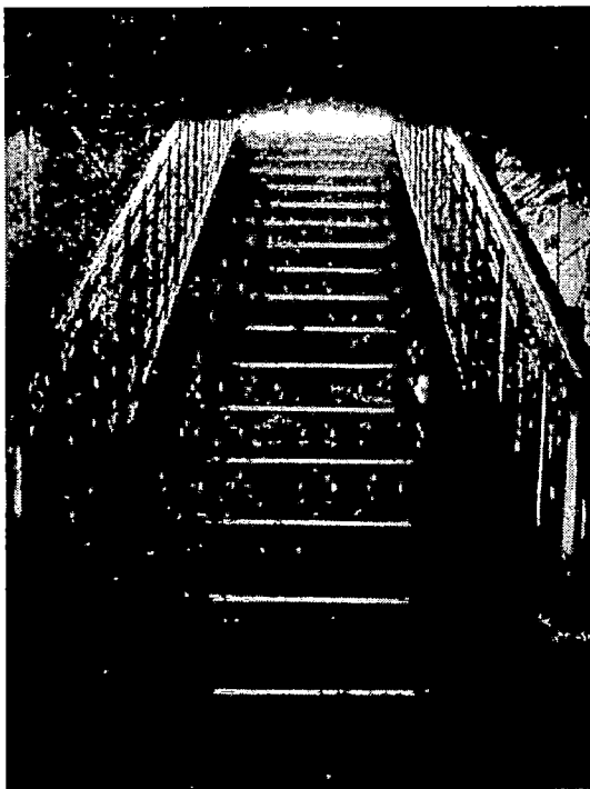
Fig 7.10: Cast iron staircase
