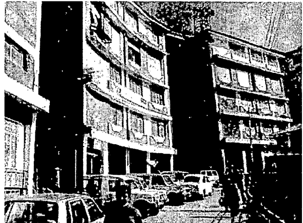
Fig 6.13: Buildings abutting the road
