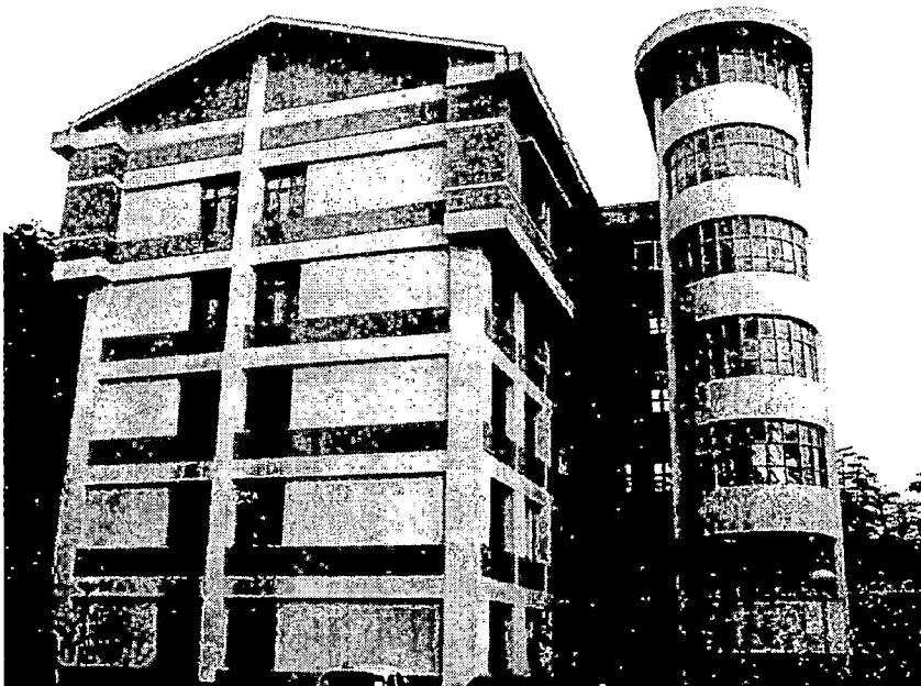
Fig 7.30: Block C of police complex
