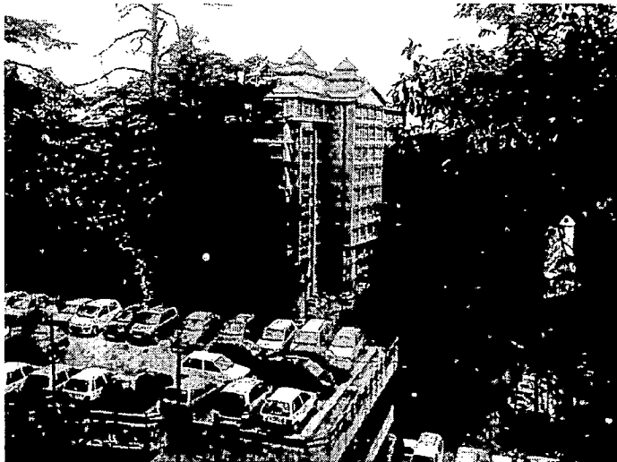
Fig 7.18: Insufficient Parking Provisions
