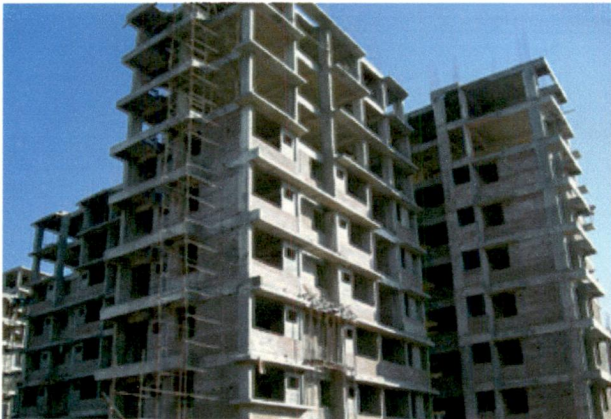
Fig 5.62: Construction Work on Site
