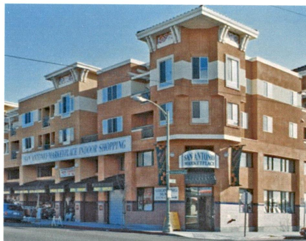
Fig 3.22: Mixed Use Development Accommodating the Local Vendors and Façade Depicting Mission Revival Style of Architecture.
