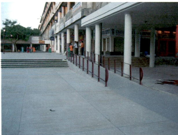
Fig.4.3: Provision of ramp for universal accessibility in Sector 17 Chandigarh.
