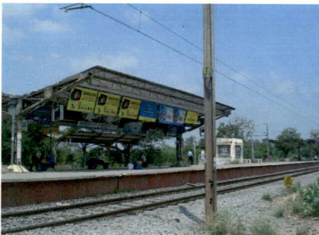
Fig 6.27: Railway Station Platforms Lacking Amenities.
