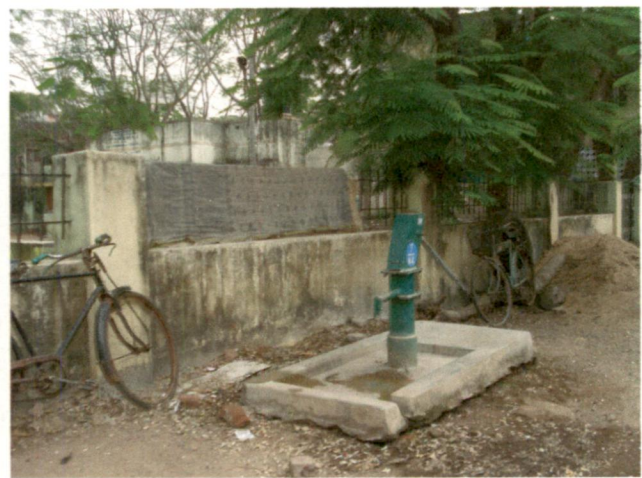
Fig 6.5: Water Supply by Hand Pumps
