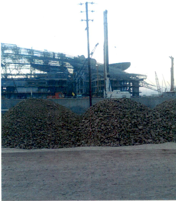
Fig 5.20: Construction Work in SIPCOT, Siruseri
