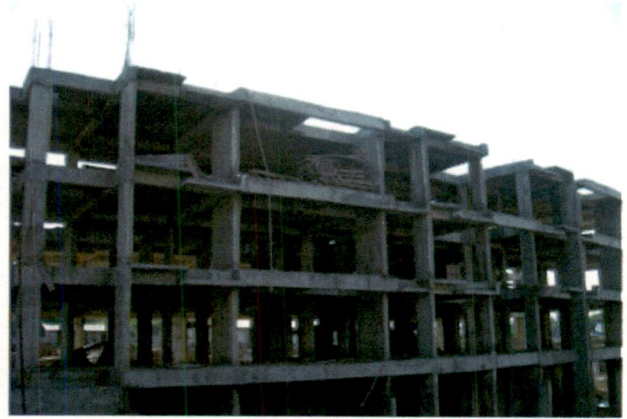
Fig 5.63: Construction Work on Site
