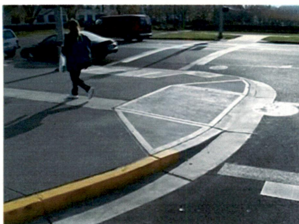
Fig 7.5: Ramp for Universal Accessibility In Salem, Oregon
