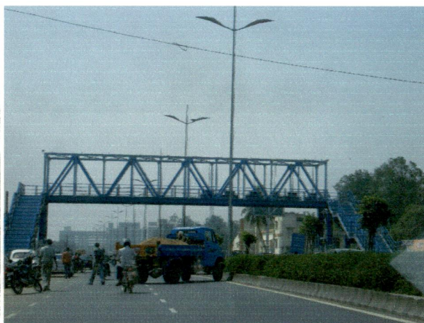
Fig 5.9: A View of the Rajiv Gandhi Salai Showing the Foot Over Bridge.
