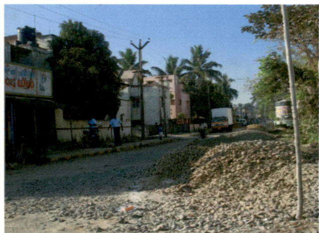
Fig 6.38: Road under Construction
