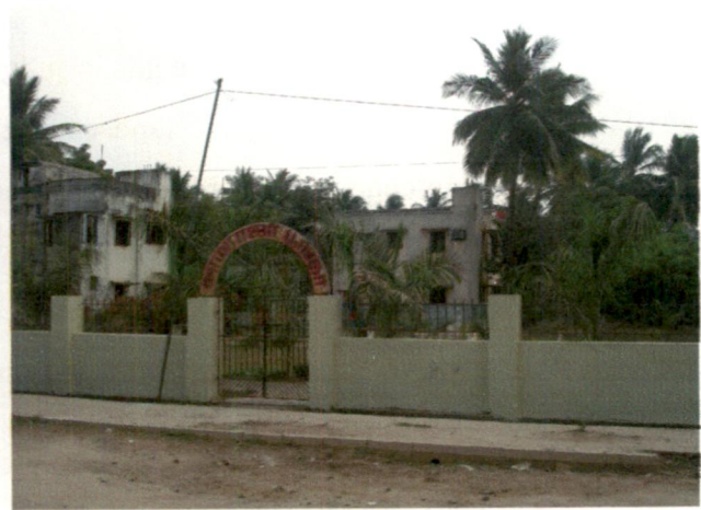
Fig 6.20: View of Kamarajar Park
