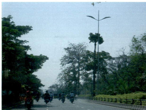
Fig 5.8: A View of the Rajiv Gandhi Salai Showing the Planter Strip and the
