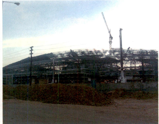
Fig 5.23: Construction Work in SIPCOT, Siruseri
