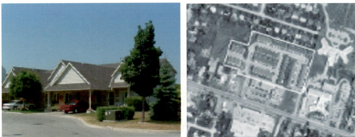
Fig 3.26: Forty Infill Townhouse Units Replace Six Singles in Grimsby to Increase Densities.
