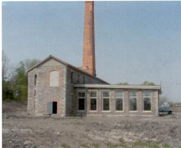
Fig 3.29: Restored Industrial Site in St. Catharines Being Converted to Office Space.
