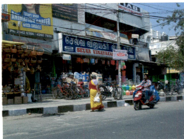
Fig 4.9: Encroached Foot Path by Shop Keepers Making the Movement of Pedestrian Difficult.
