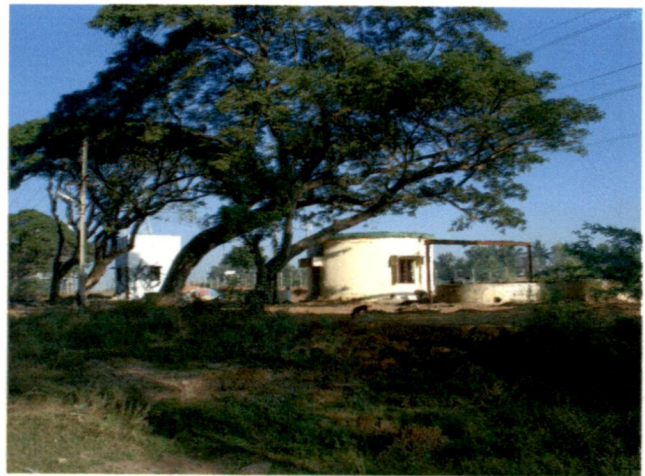
Fig 6.9: Pumping Station and Oxidation Pond
