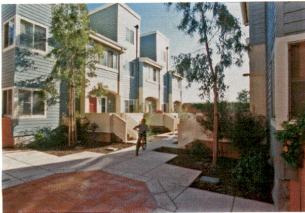
Fig 3.19: A Central Courtyard above the Parking Garage.
