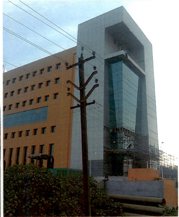
Fig 5.21: Office Complex SIPCOT, Siruseri
