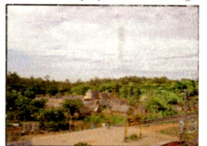
Development of slum along the railway track
