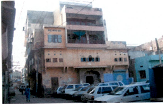
Fig 5.11: Addition of extra floors and change in old fabric
