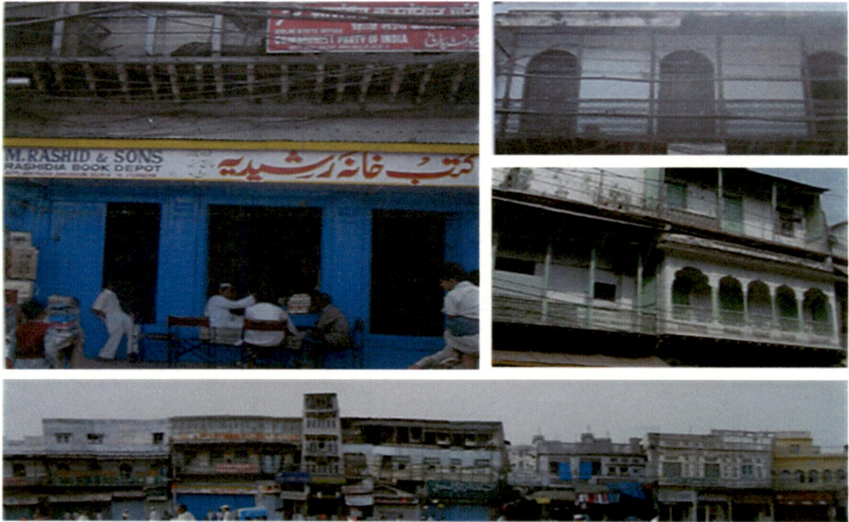
Fig 3.1: Some buildings worth preserving
