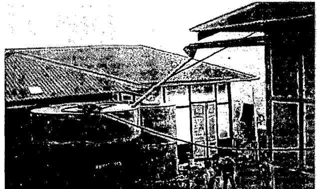
The Mizoram government took up rainwater harvesting under its public water supply programmes in 1986. As a policy, it is replacing all thatch roofs with galvanised sheet roofs to promote rooftop water harvesting.
