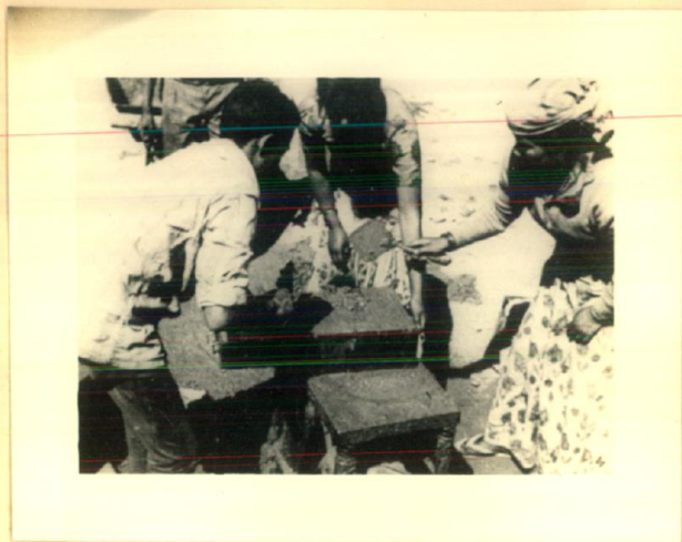
13. CEMENT HOLLOW BLOCK CAST OVER PLATFORM VIBRATOR
