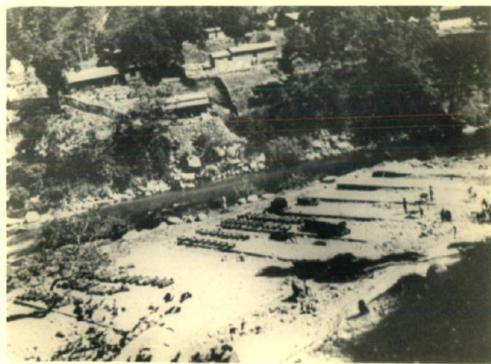
VIEW OF COLLAR BEAM CASTING YARD
