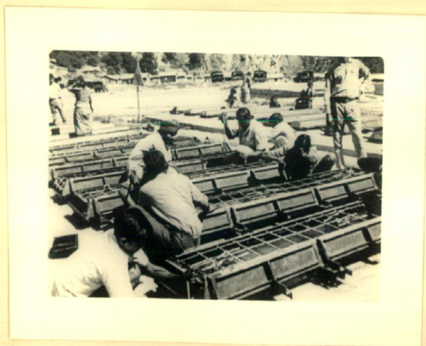
TROUGH REINFORCEMENT PLACED IN STEEL MOULDS
