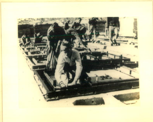
STEEL MOULDS FOR PANELS UNDER ASSEMBLY
