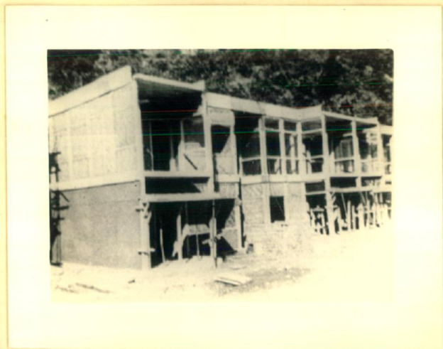
VIEW OF VARIOUS STAGES OF LATH PLASTER AS AN ALTERNATIVE TO HOLLOW BLOCK INFILL.
