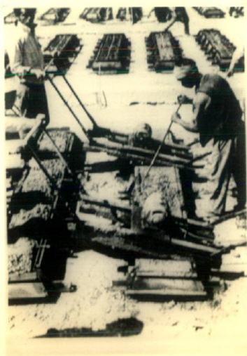
CASTING OF TROUGH IN PROGRESS (EXTERNAL VIBRATOR IN USE)
