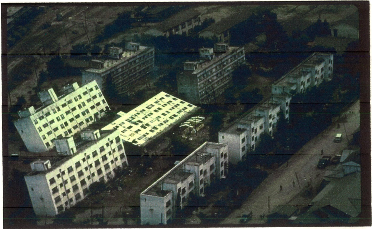
Fig. 2.4 Tilting of buildings at Kawagishi-Cho, Niigata Earthquake, 1964 ( www.ce.washington.edu/~liquefaction/selectpiclique/nigata64/tiltedbuilding.jpg )
