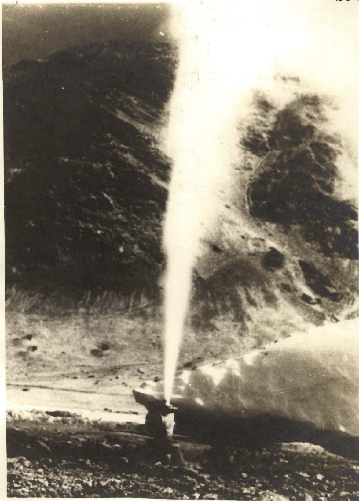
FIG. VI-13 Steam and Water Mixture Blowing from a Drill Hole Puga Geothermal Field
