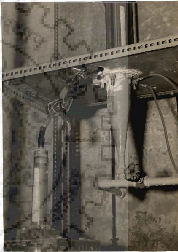
FIG.5.4 PHOTOGRAPH SHOWING SOLIDS DISCHARGE AND SAMPLING ARRANGEMENT.
