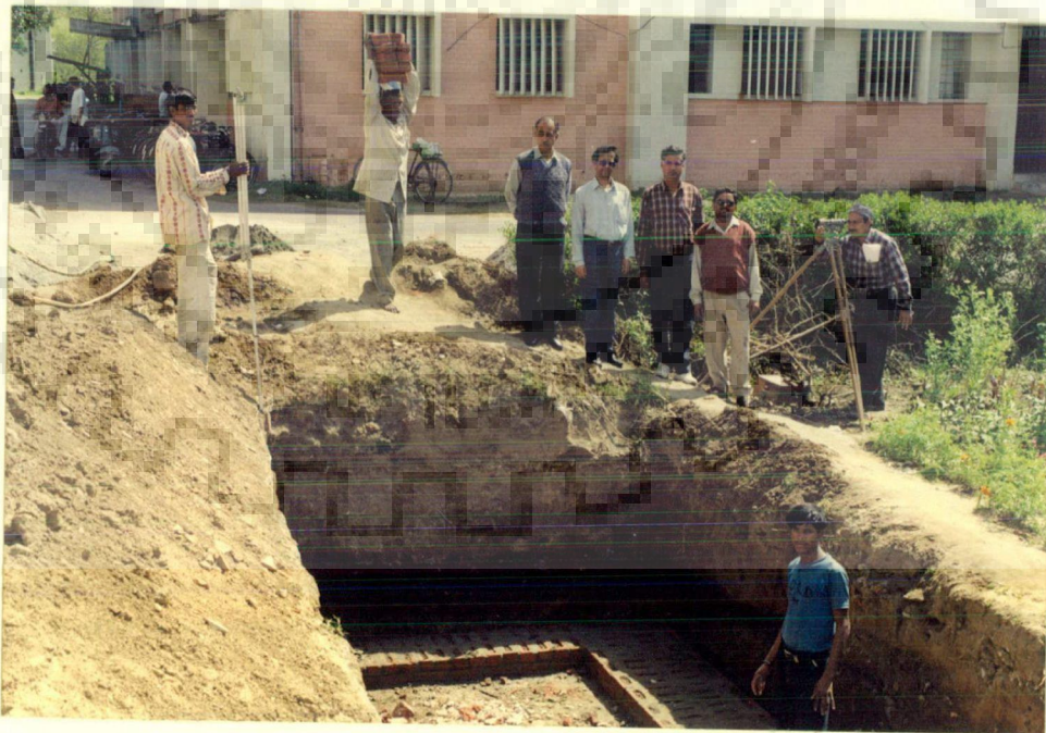
Plate A3.1b: CONSTRUCTION OF WATER STORAGE TANK OUT SIDE THE BUILDING
