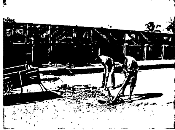
Fig 8.06: Maintenance of Broken Roads
