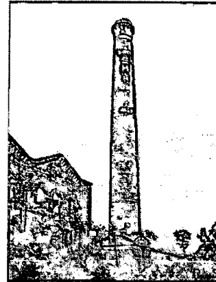
1.2 Dilapidated non-functioning textile mill
