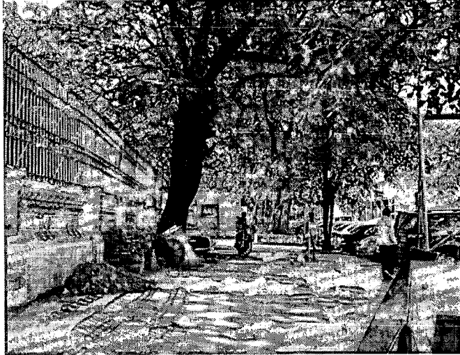
6.20 The existing pavement condition
