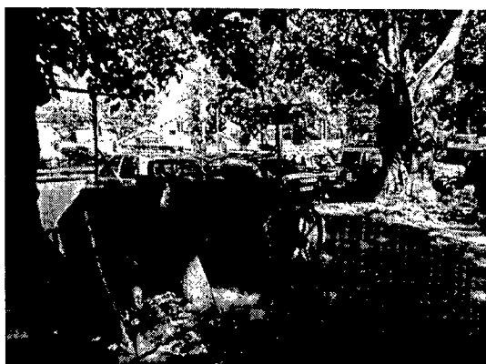
4.34: Same footpaths under bad conditions on other days
