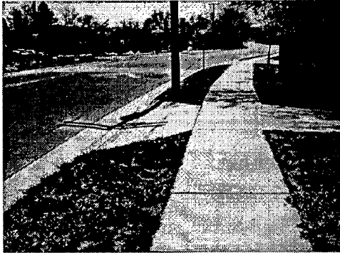
Fig. 2.21: Curb ramp in sidewalk, Chicago
