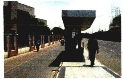
Fig. 5.46: Well-planned sidewalk, Canal Bund Road Source: By Author
