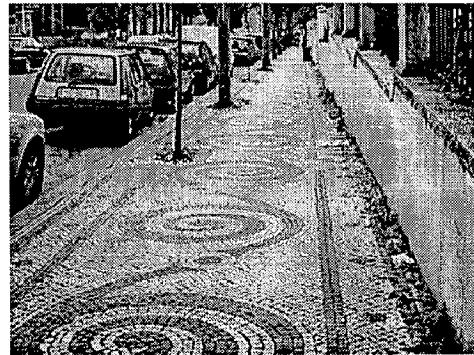
Fig. 2.26: Paved sidewalk in Portugal
