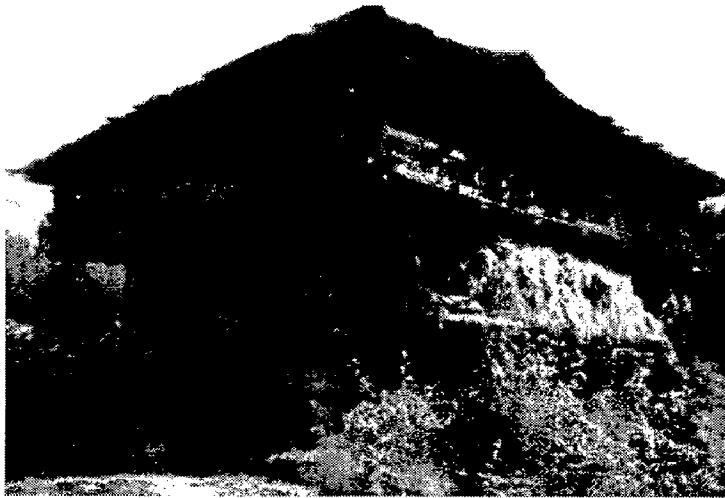
Figure 5.1 Traditional house in Kinnaur with Kath Kunni construction
