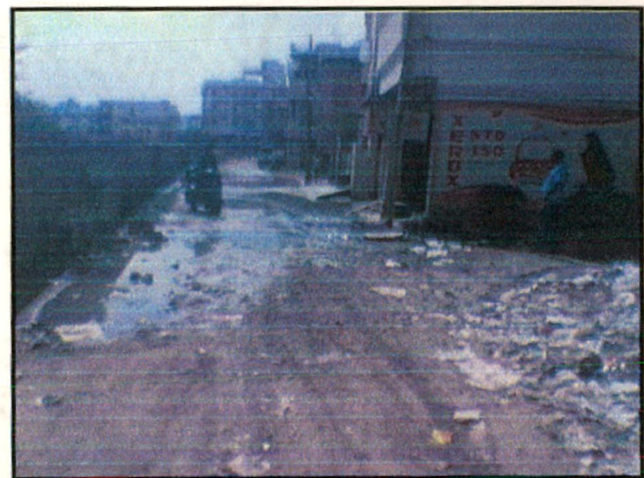
Fig. 7.4. Overflow of drains
