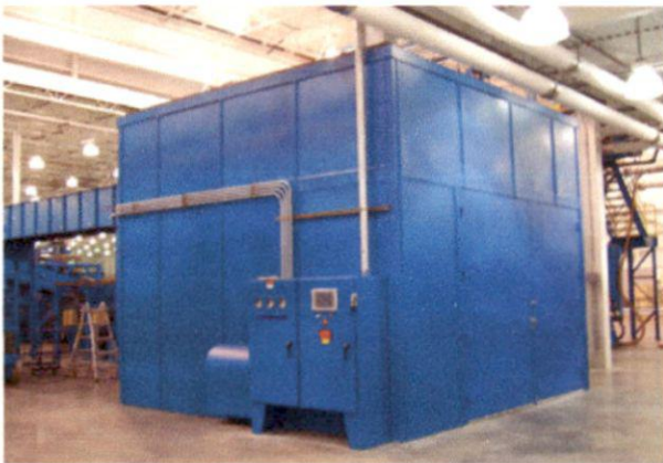
Figure 5.25: Sound Enclosure System for HVAC and Power Generators
