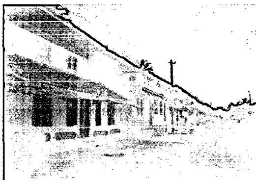
Figure 5.40-View of Kizhakkencherry agraharam from south
