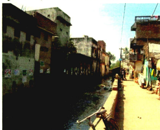
Figure 5.1: The road along the main drain Source: Primary survey by author
