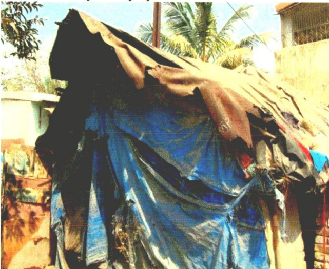
Figure 5.15: A hut made out of polythene Source: Primary survey by author
