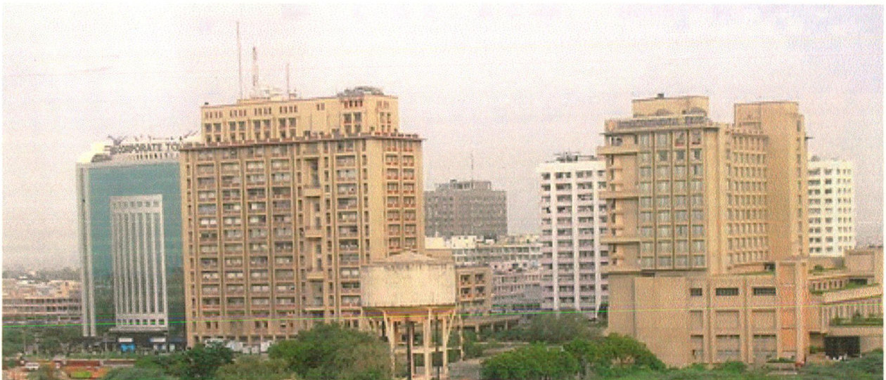
Fig 4.3: Offices located in N.P.
