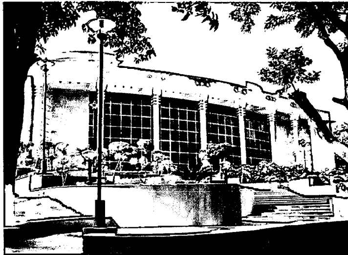
Fig 3.4: Front façade of the Central Library
