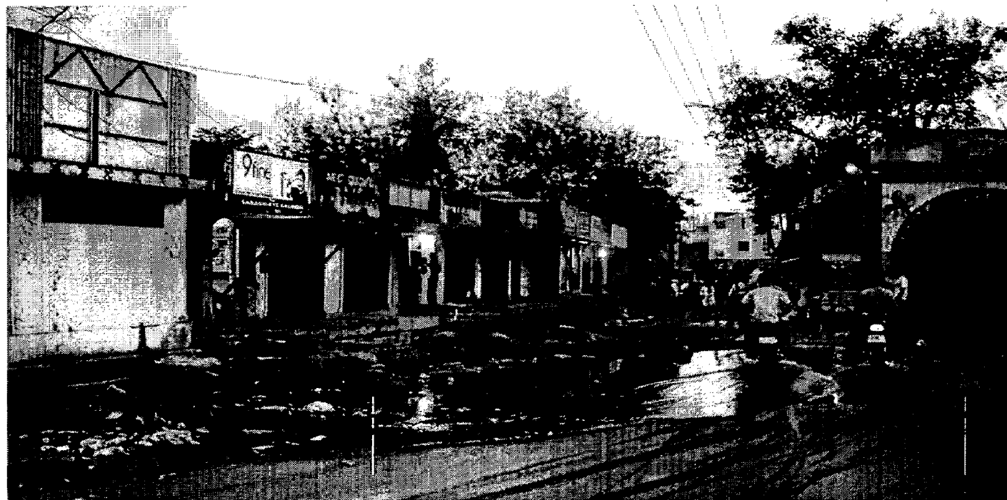
Fig.6.13. Overflow of sewage into roads creates bad sanitary conditions.
