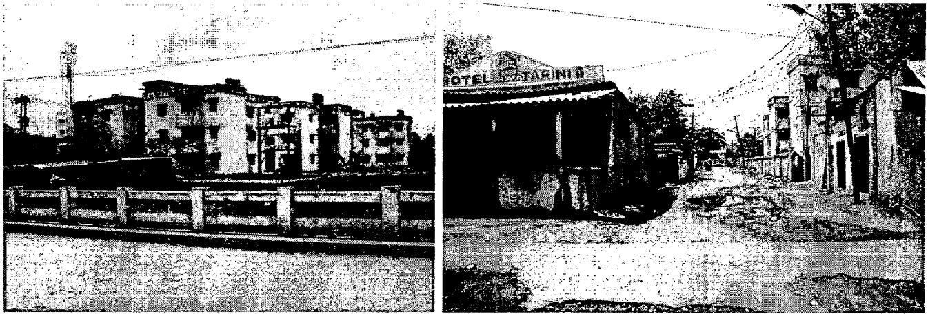
Fig.7.5. Residential structures in the residential Zone towards the east
