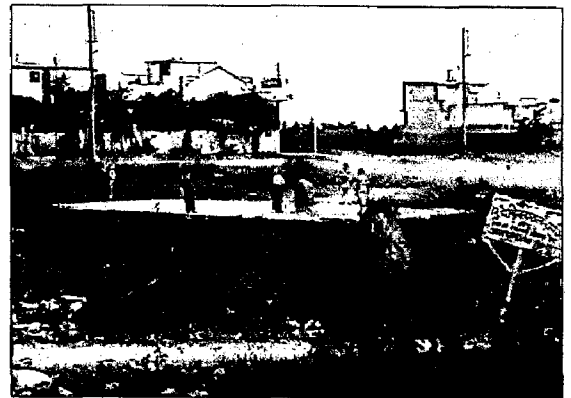
Fig 9.13 Septic tank situated in the park.
