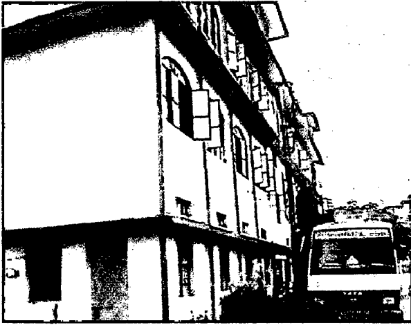
Fig 9.27 school building in sarvdharm colony
