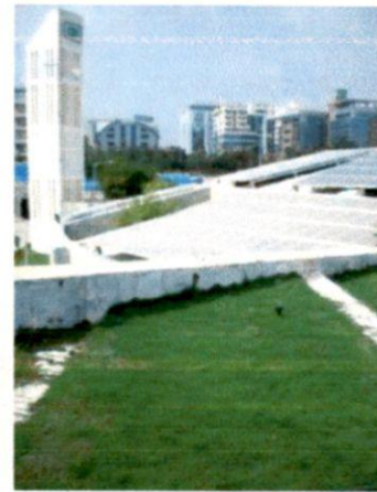
Figure 3.9 view of Green roof
