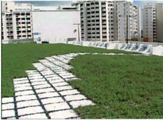
Figure 2.3 Aesthetic Potential of Extensive Green Roof Tray Systems
