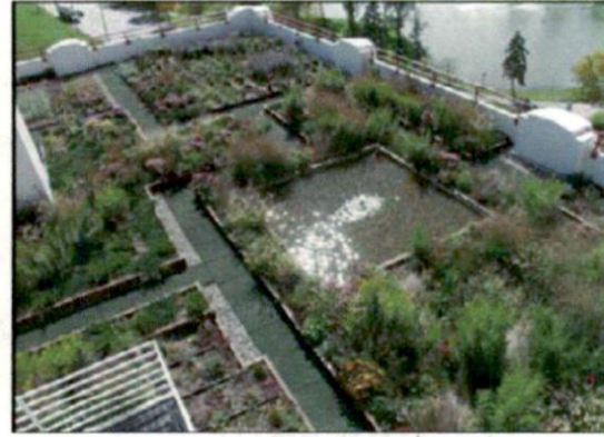
Figure 2.4 Typical Extensive Green Roof Tray System in India
