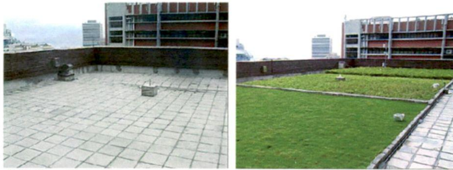
a) Before Retrofit
