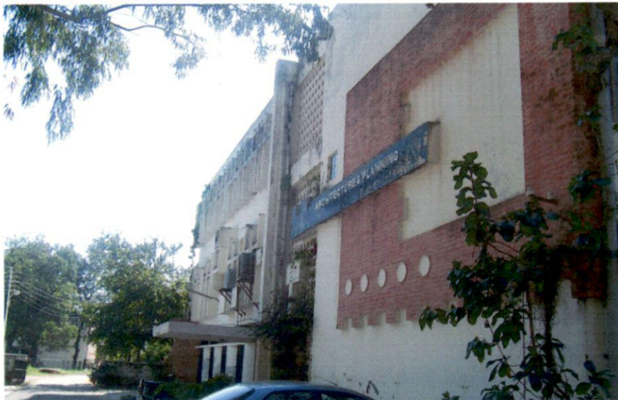
Figure 6.1 Department of Architecture and Planning
