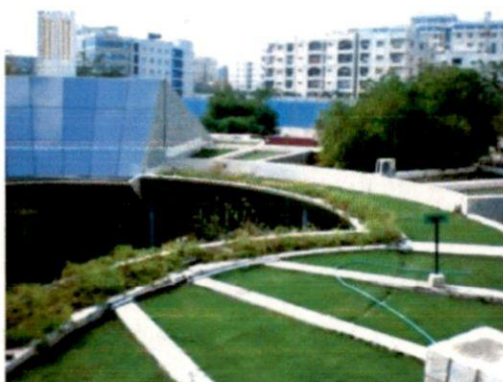
Figure3.8 Extensive green roofs
