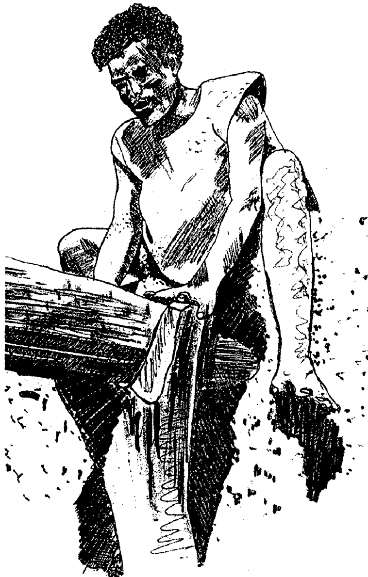
FIG: 3.3. RIDGE BEAM BEING PLACED ON A FORKED UPRIGHT
