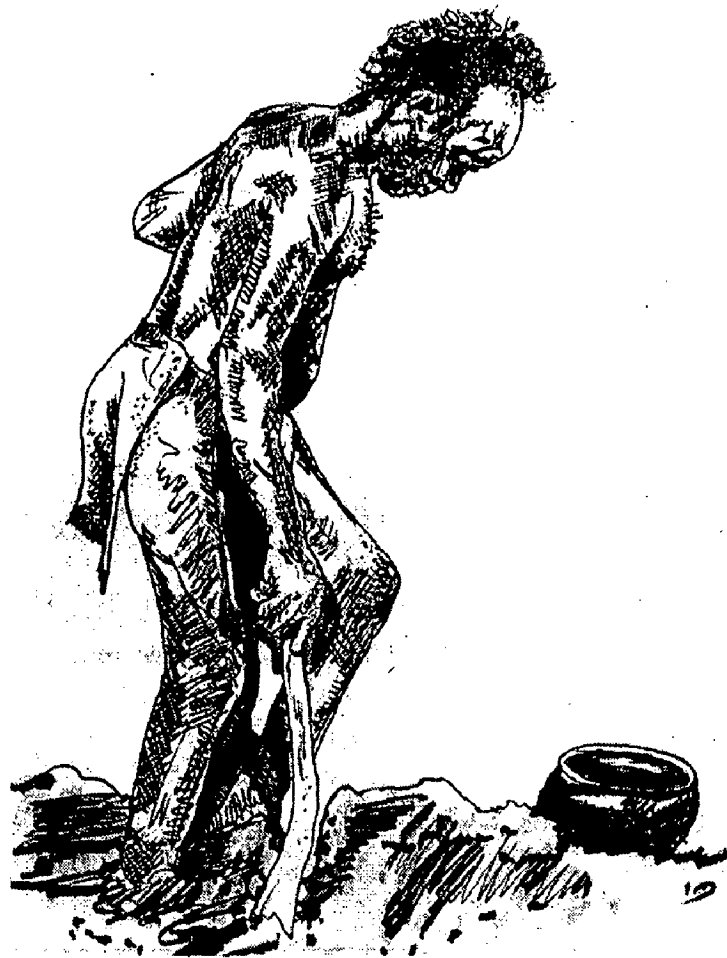
KNEEDING OF ARGILLACEOUS CLAY WITH WATER IN PIT, FOR HOUSE CONSTRUCTION, NEAR TO THE HOUSE CONSTRUCTION SITE.
