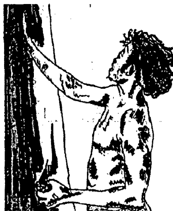
BEDAUBING OF MUD WALL WITH DISTRIBUTED MUD PLASTER, MIXED WITH COW DUNG.
