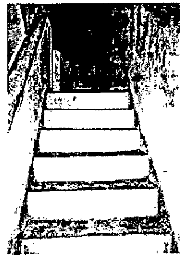
Fig 5.5.20 View of staircase
