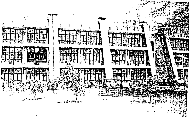
3. SOUTH FAÇADE DEPICTING THE USE OF SOLAR PANELS
