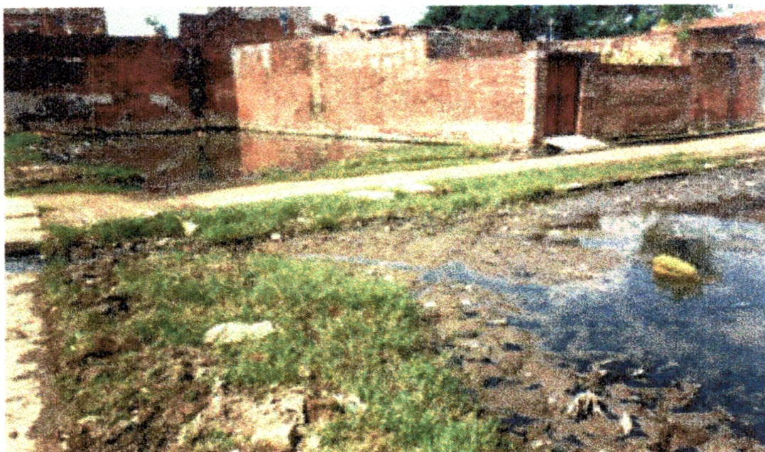
Water logging in vacant plots
