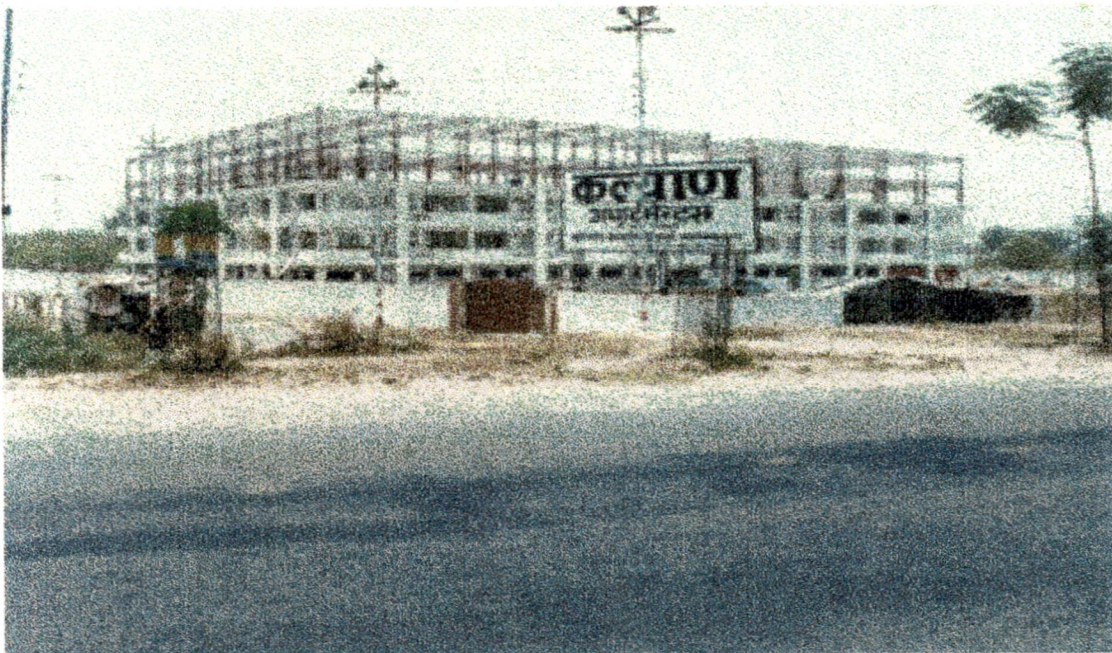
New construction techniques
