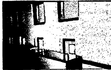
Windows from inside (Office space)
