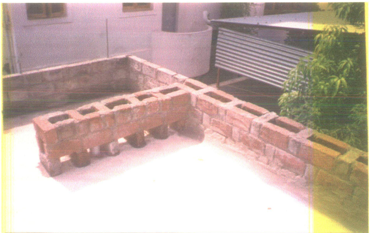
Fig. 4.37 View Shows The Wall Construction Technique
