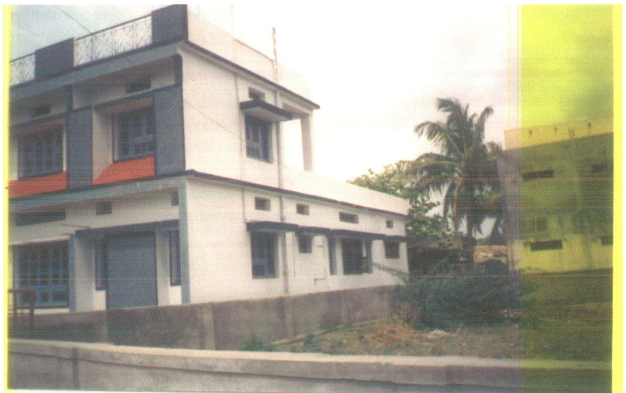
Fig. 4.16 South-West View of Hebbal House
