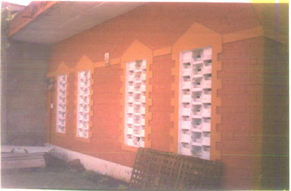
Fig. 4.34 Front View Showing Windows of S.V. Bakshi House
