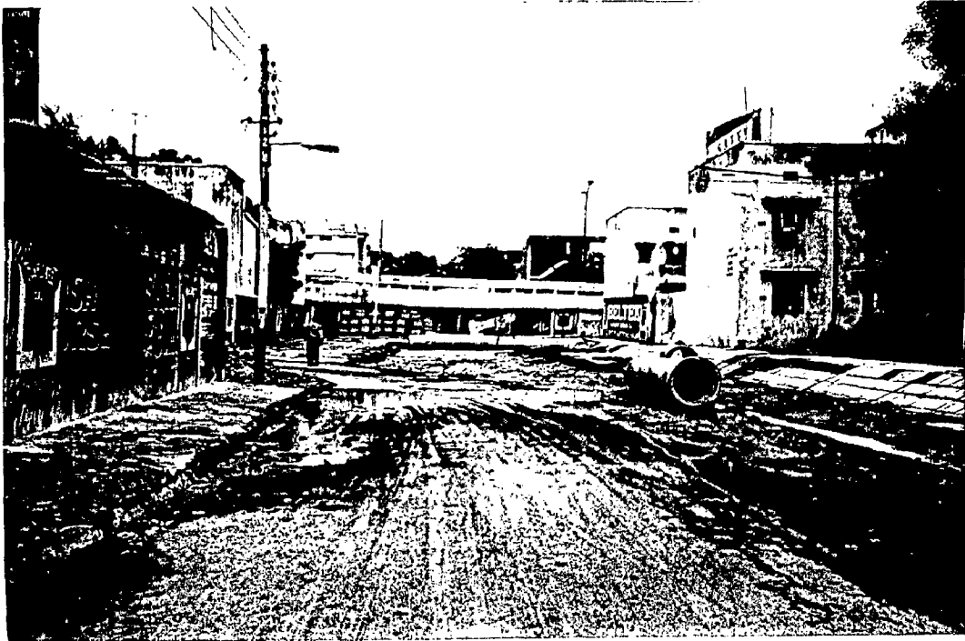
ONE OF THE FEW WATER LOGGED ROADS
