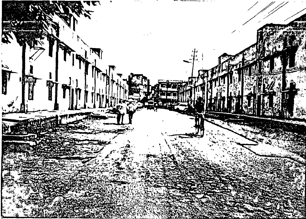
DEVELOPMENT - DOUBLE STOREY FLATS WITH WELL MAINTAINED WIDE ROADS
