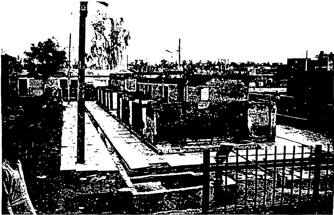
M.C.D. TOILETS - IN THE STATE OF RUINS
