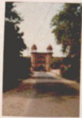
ENTRANCE FROM G.T. ROAD.
