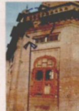
MISSING/BROKEN CHAJJAS
