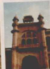
MONUMENTAL SCALE TYPICAL ARCHES, JHARKHAS.
