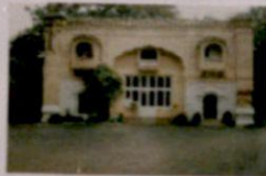
UNATTENDED FACADES : PALACE
