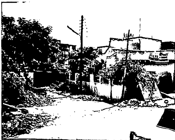
E. CONSTRUCTION DEBRIS
