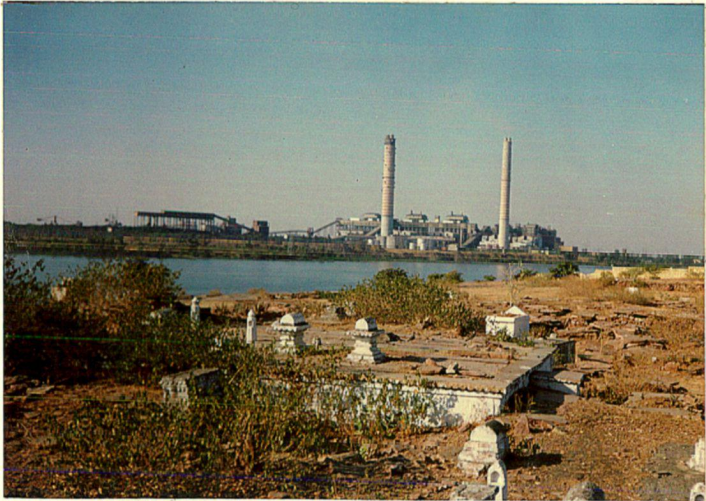
4. KOTA THERMAL POWER PLANT AND RESERVOIR CREATED BY THE BARRAGE ON RIVER CHAMBAL.
