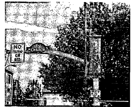
Figure 36 Street name sign on mast arm
