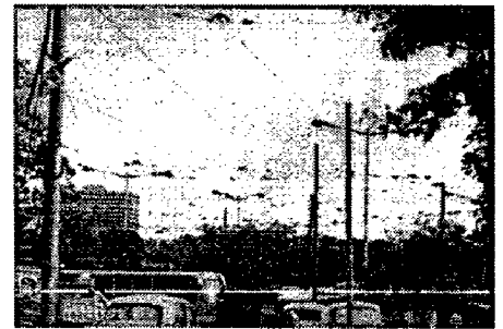
Figure 94 Well maintained OHE wire
