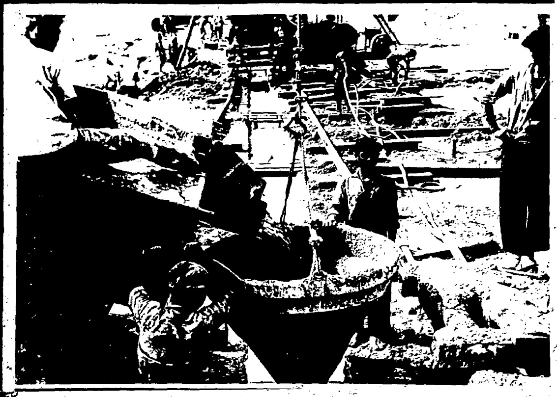
Concreting by Tremie
