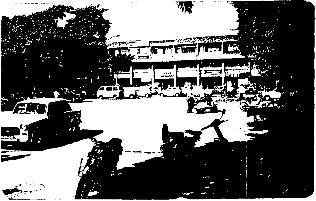
FIG.4.4 SHOPPING MARKET OF A SECTOR CARE HAS BEEN TAKEN TO PROVIDE BIG CENTRAL AREA FOR PARKING AND OTHER ACTIVITIES.
