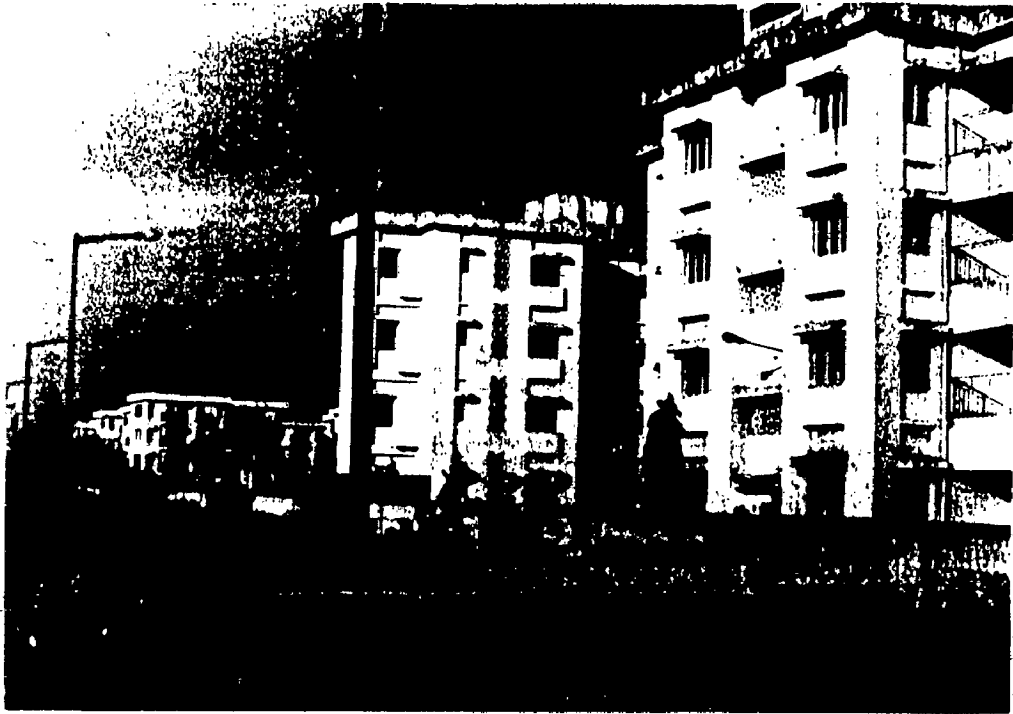
Multistorey Development in Salt Lake
