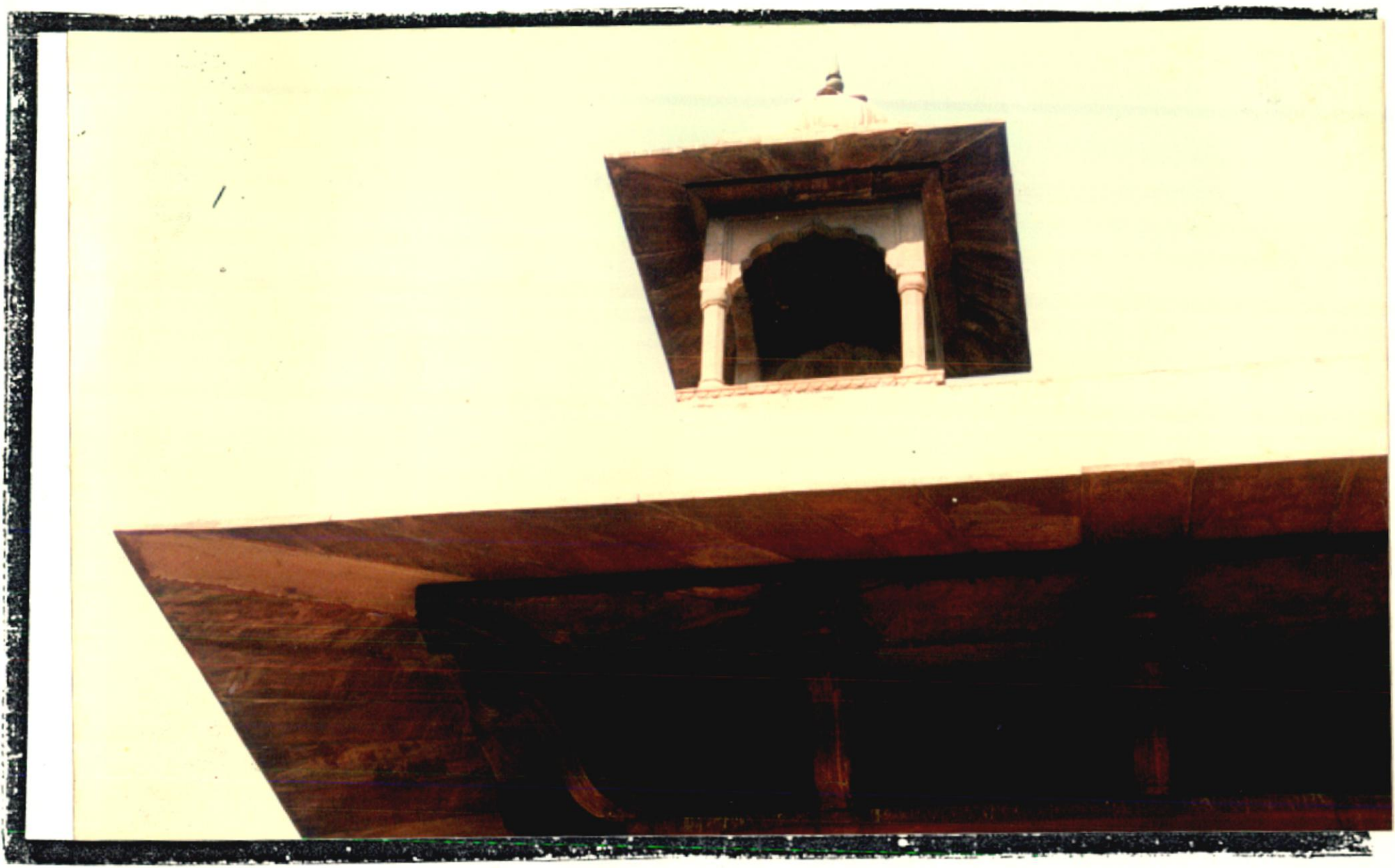
Location : Roof of Diwane Aam, Lal - Quila.
